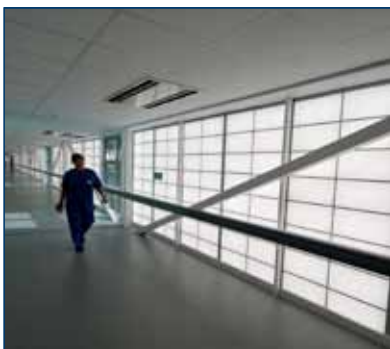
KALWALL WALKWAY AT QUEEN ELIZABETH HOSPITAL BIRMINGHAM CONNECTS ONCOLOGY WITH THE MAIN BUILDING.
