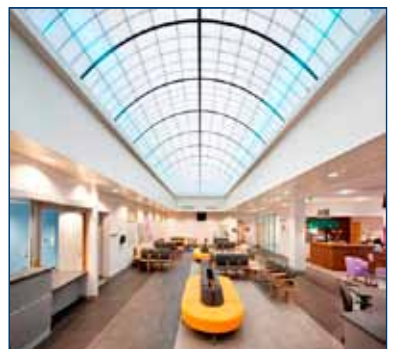
THE KALWALL CURVED ROOF OF LOXFORD POLYCLINIC IN ILFORD, EAST LONDON IS 17M LONG X 5.7M WIDE
