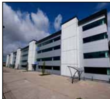
THESE WAREHOUSES AT LONDON'S HEATHROW AIRPORT HAVE THEIR STAIRCASES ENCASED IN KALWALL
